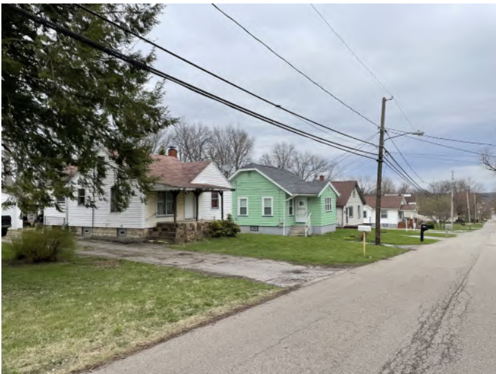
Valacamp Avenue - Looking East
